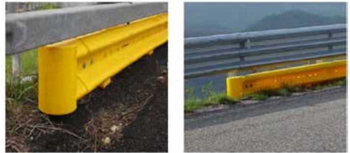
Figure 8: Connect DR46 MBA end modules
