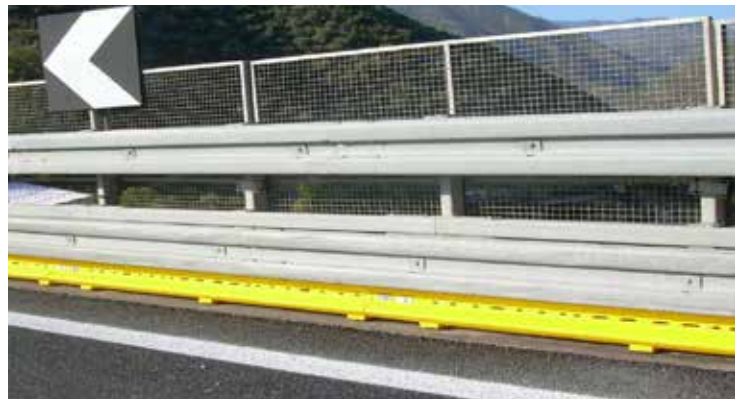
Figure 5: Approved custom installation using spacers
