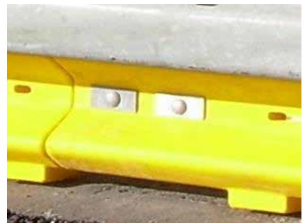
Figure 3: Connection between modules
