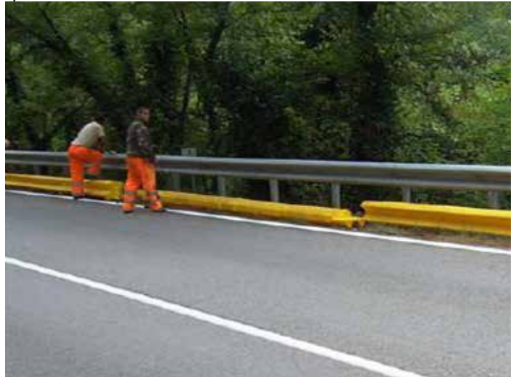
Figure 4: Position the DR46 MBA modules where they will be installed
