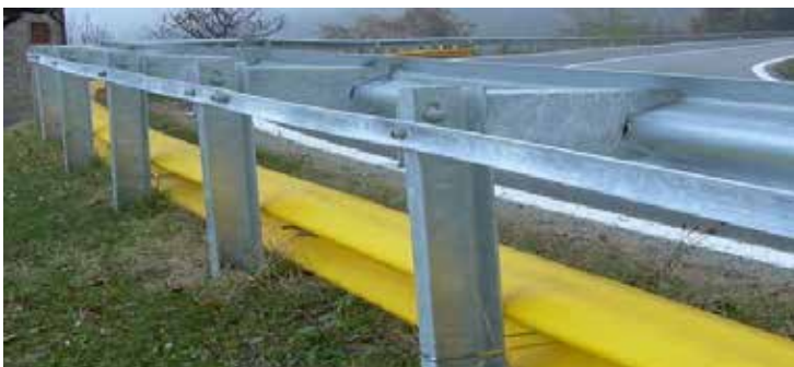
Figure 7: Position and attach the DR46 modules
